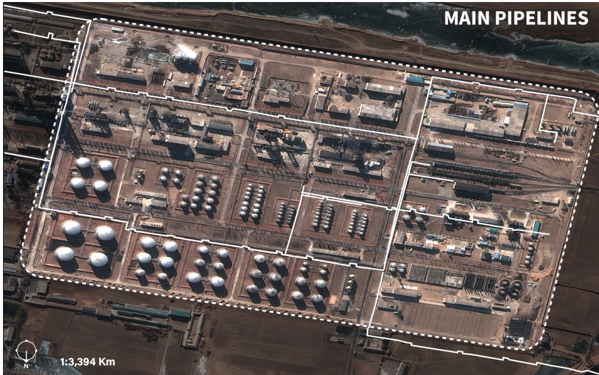
Figure 13: Main Pipe Tracks Throughout the Site
