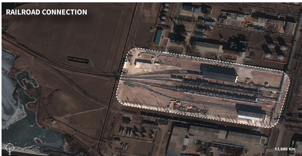
Figure 15: Rail Loading/Offloading Yard
