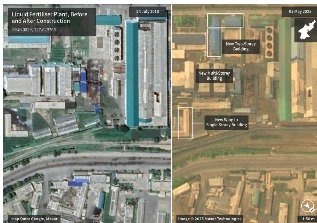
Figure 22: Liquid Fertiliser Plant, Before and After Construction
