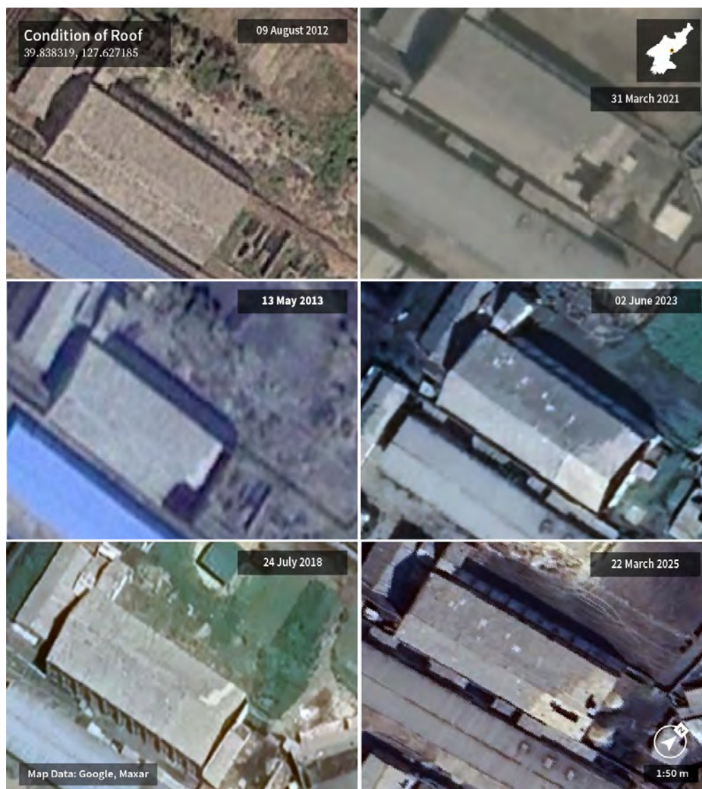
Figure 27: Condition of Roof
