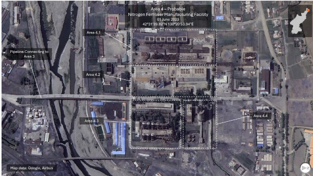
Figure 12: Area 4: Probable Nitrogen Fertiliser Manufacturing Facility
