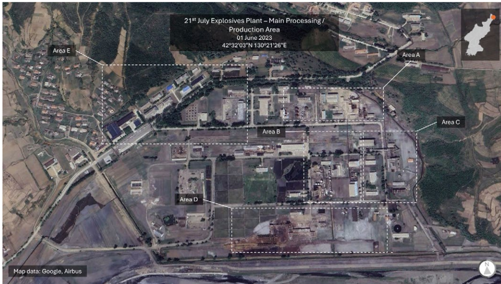
Figure 23: 21 st July Explosives Plant Main Processing and Production Area
