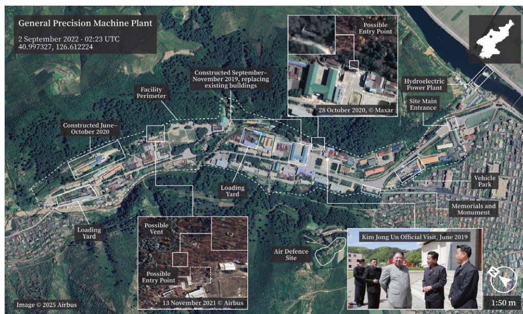
Figure 4: GPMP, Area Overview
