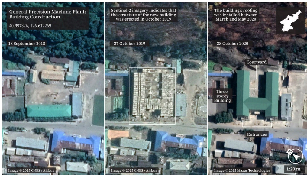
Figure 5: Construction of H-Shaped Building at the General Precision Machine Plant, 2018–2020
